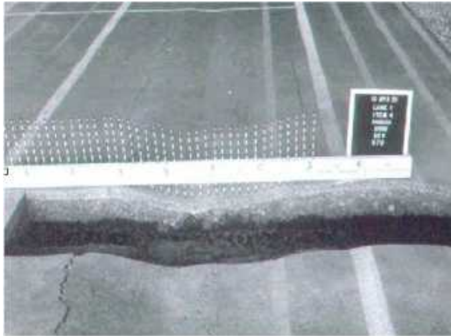
Figure 1-6. Normal rutting.
